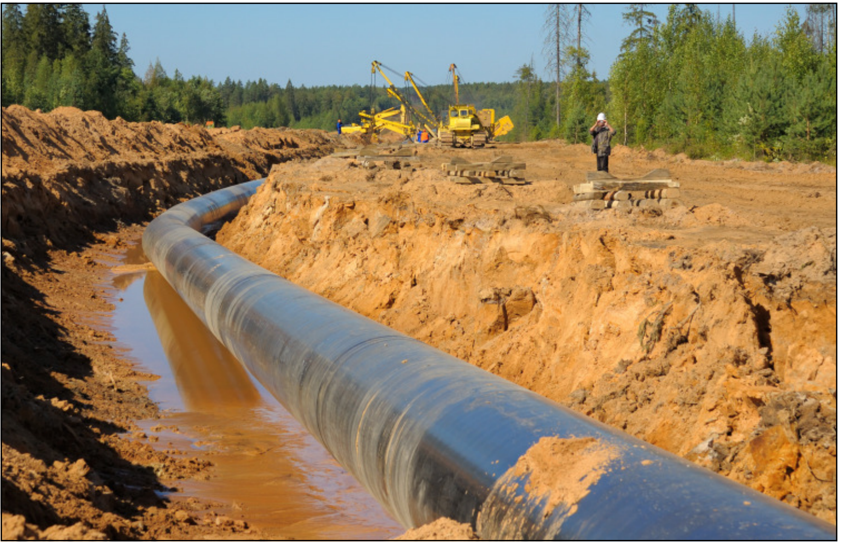
A 42-inch pipeline being built in Pennsylvania
